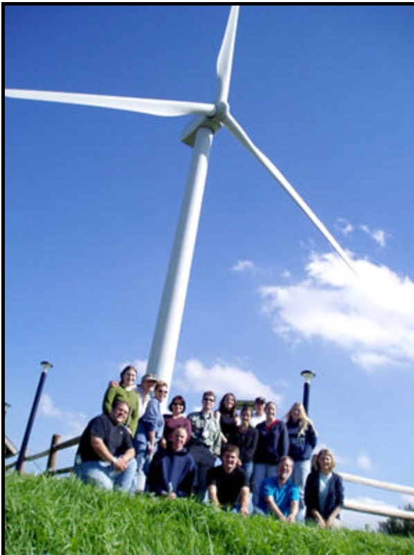
Allegheny purchases about 1/4 of the annual electricity generated by one of these wind turbines.
