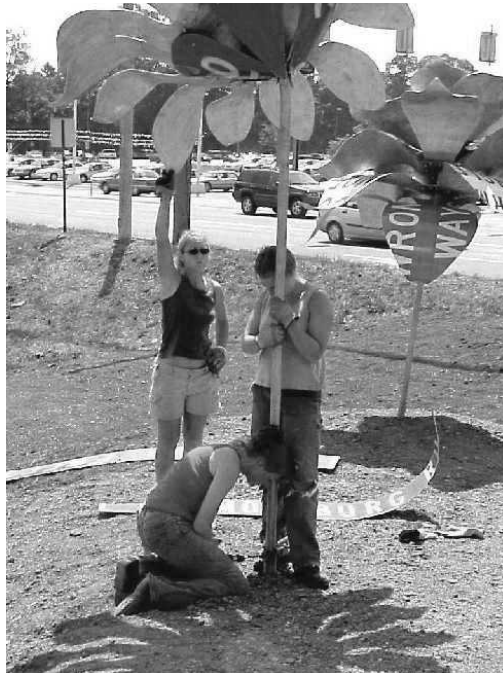
As part of phase one, students installed "flowers" made of street signs at the intersection of Routes 322 and 102.
